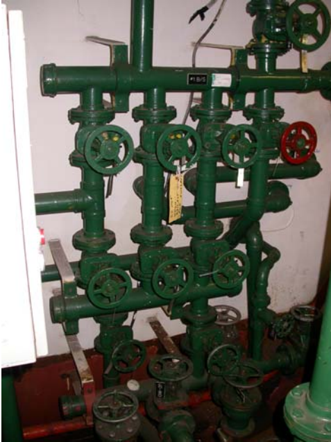
Bilge/ballast manifold
